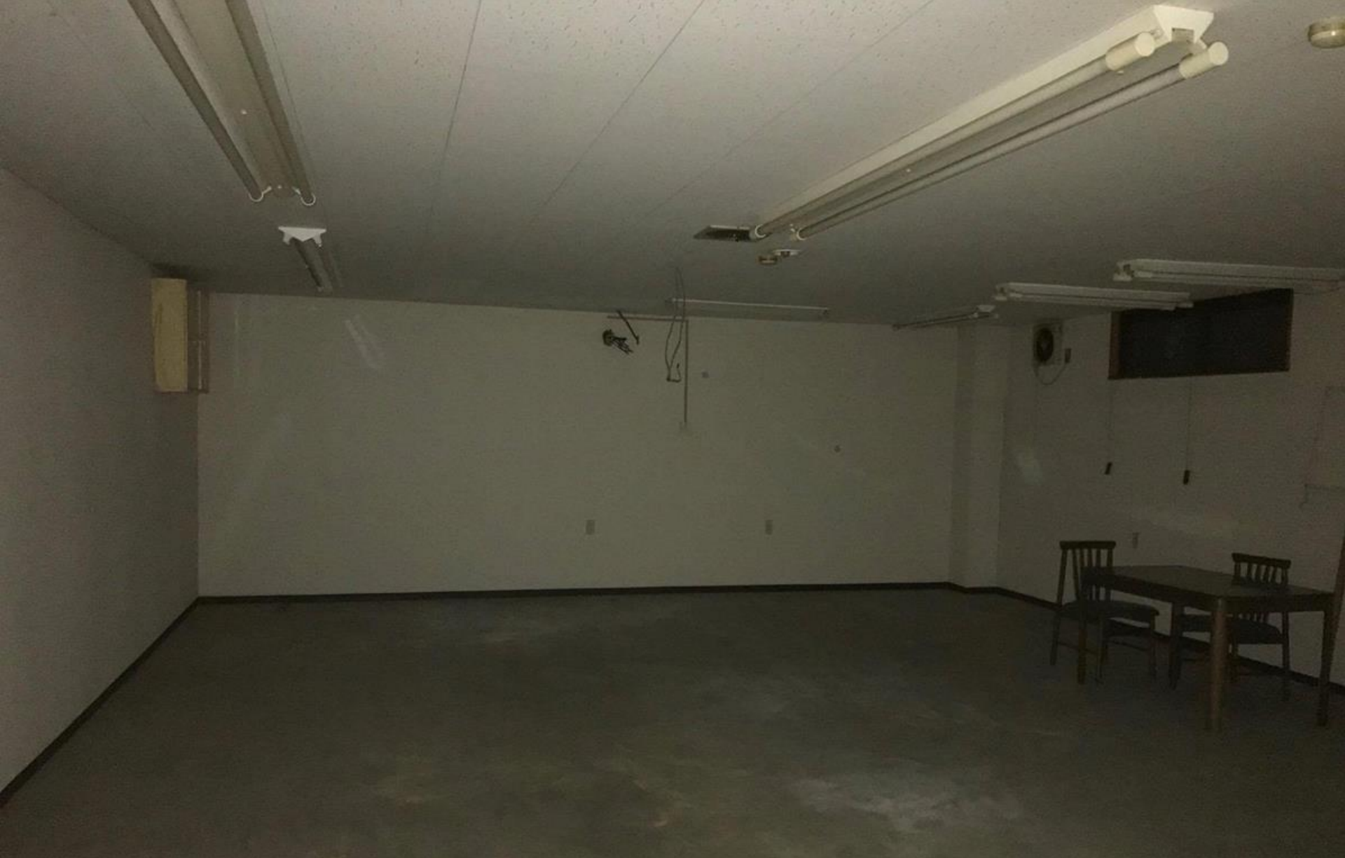
Uruwashi Building, 2 nd floor
